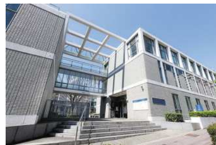
Kobe Yamate Campus Building No. 3
